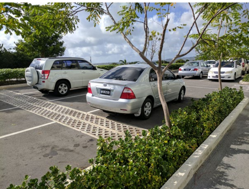
➤ Parking designed to address stormwater, The Pine
