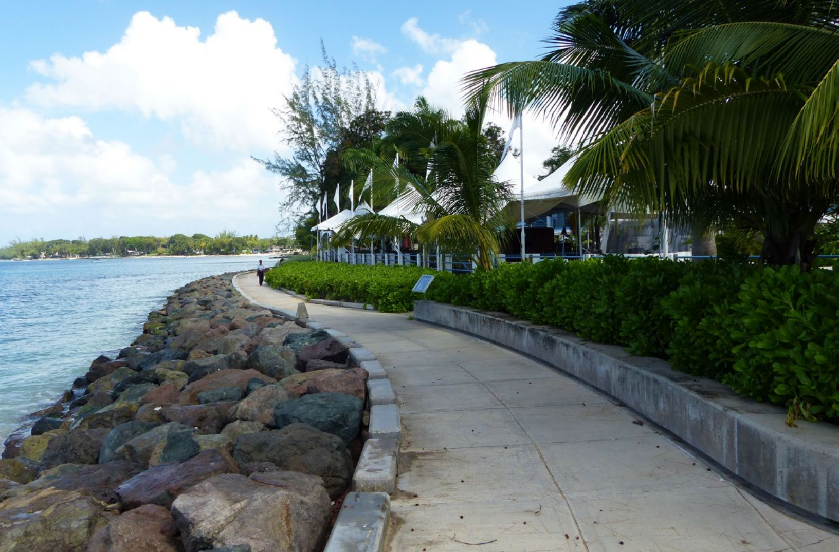
➤ Reinforced shoreline and boardwalk, Holetown, St. James
