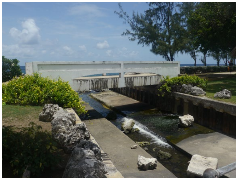
➤ Stormwater channel, Trevor's Way, Bridgetown
