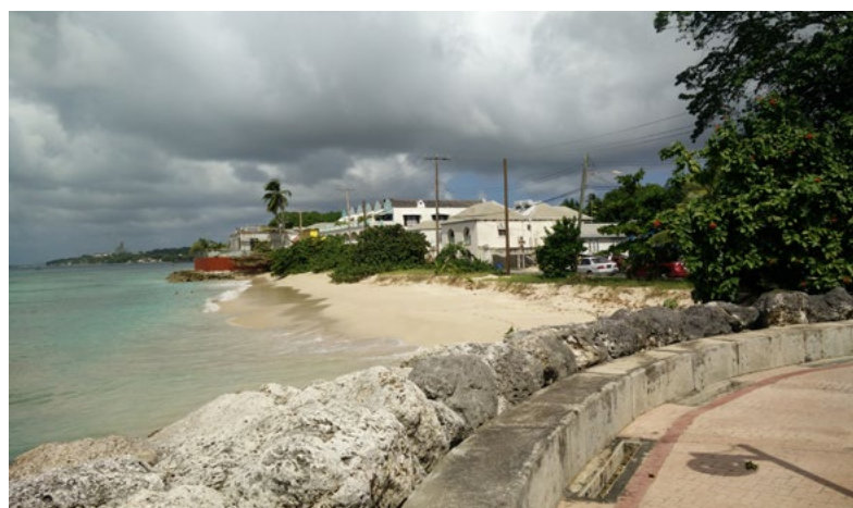
> Coastal erosion, Sand Street, Speightstown
