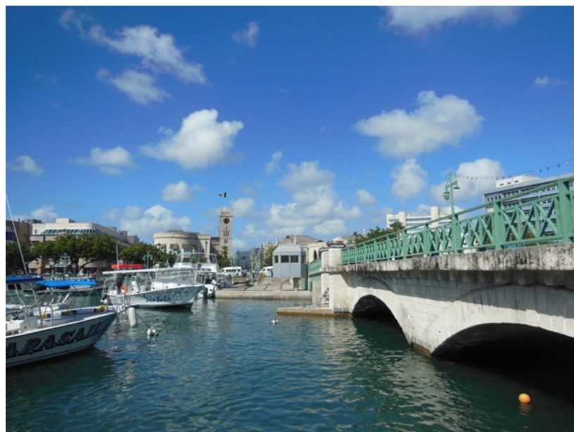
> South side of the Careenage (Bridge House)
