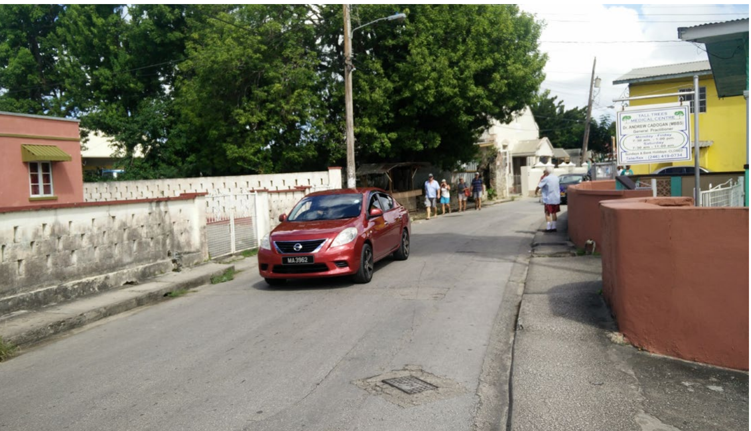
➤ Existing sidewalks are intermittent along Church Street
