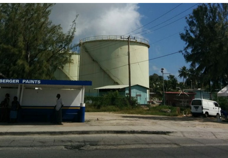
➤ Disused fuel storage tanks, Oistins, Christ Church
